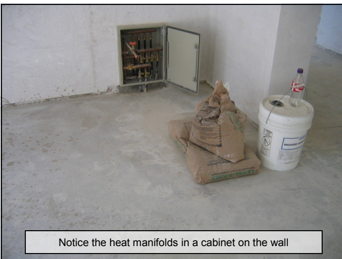
Level-Right over radiant tubing
