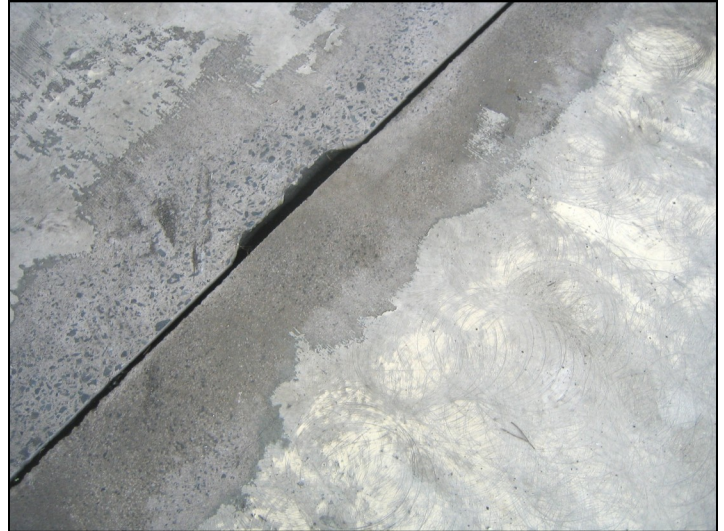
Pictures of the old epoxy floor.
